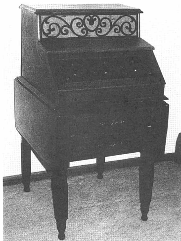
Wolper model RS5; slant-front radio in very deep case, with stepped-back enclosed speaker; mid-1920s. The radio is sitting on a separate table (Paul Johnson).
